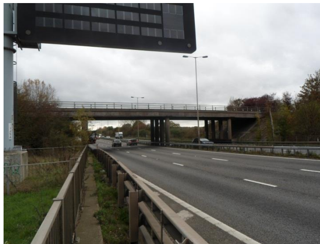
Figure 2 View of the existing Monkey Island Bridge
