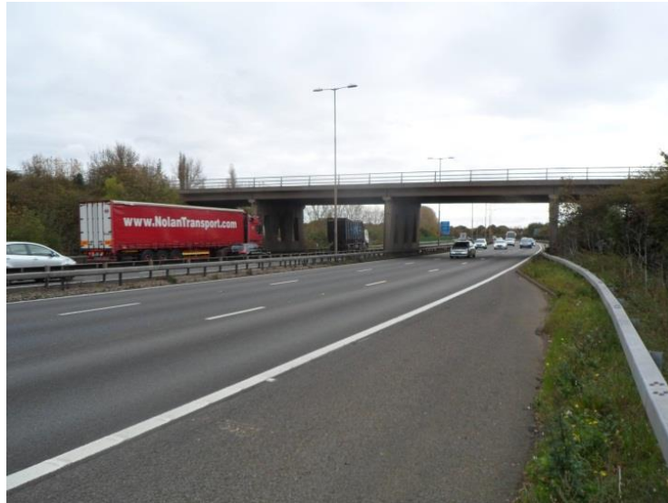
Figure 36 View of the existing Riding Court bridge
