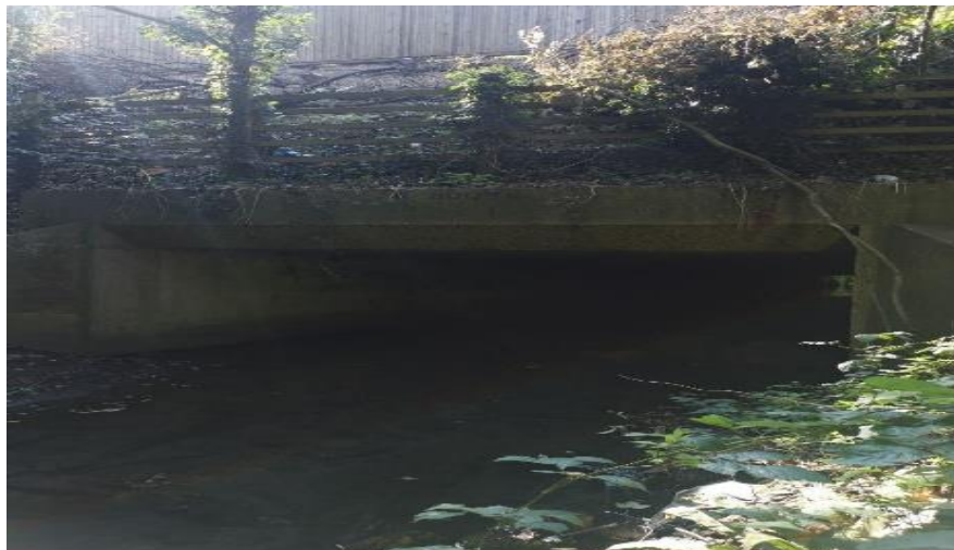
Figure 32 View of Railway culvert from the North
