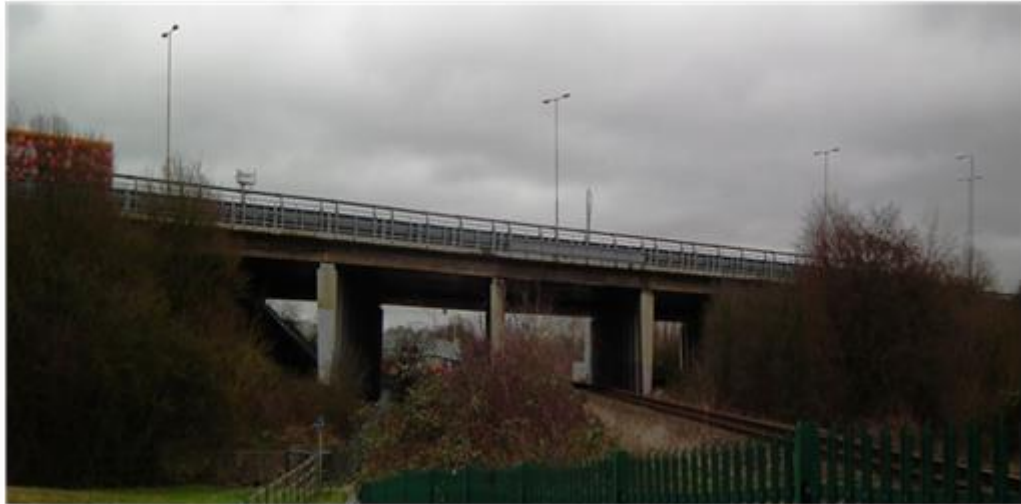
Figure 33 View of Windsor Branch Railway Bridge from the South
