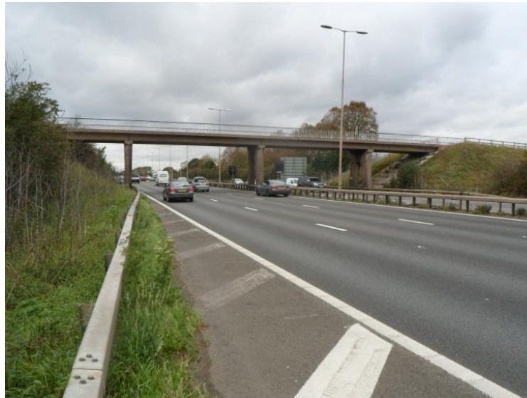
Figure 29 View of the existing Oldway Lane bridge
