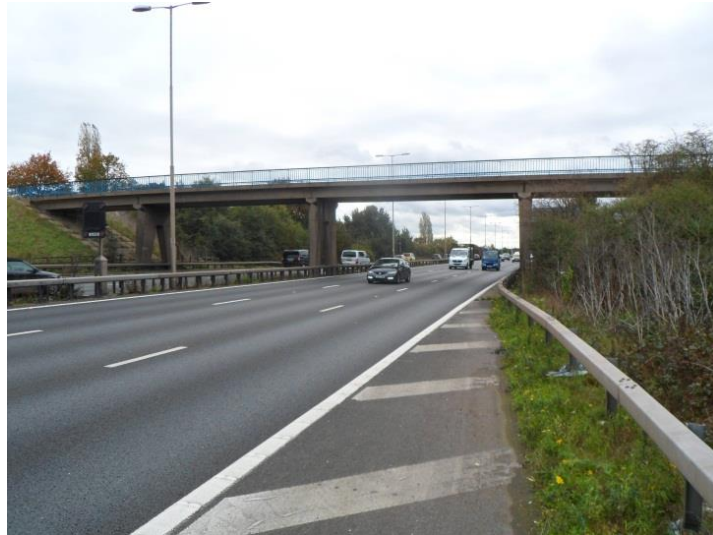
Figure 35 View of the existing Recreation Ground bridge
