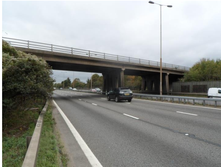
Figure 4 View of the existing Marsh Lane bridge
