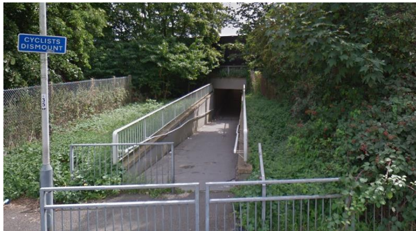
Figure 8 Sipson Road subway from the north
