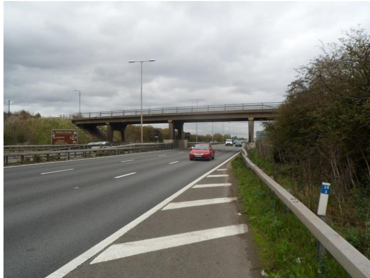
Figure 30 View of the existing Wood Lane bridge
