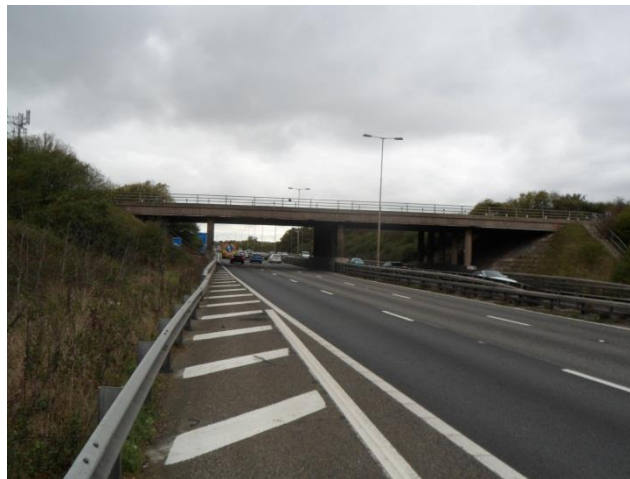
Figure 1 View of the existing Ascot Road Bridge
