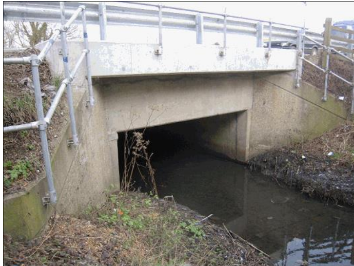
Figure 31 View of the southern of Chalvey culvert
