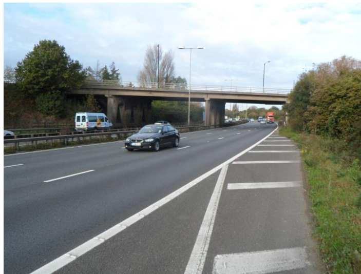
Figure 6 View of the existing Datchet Road bridge
