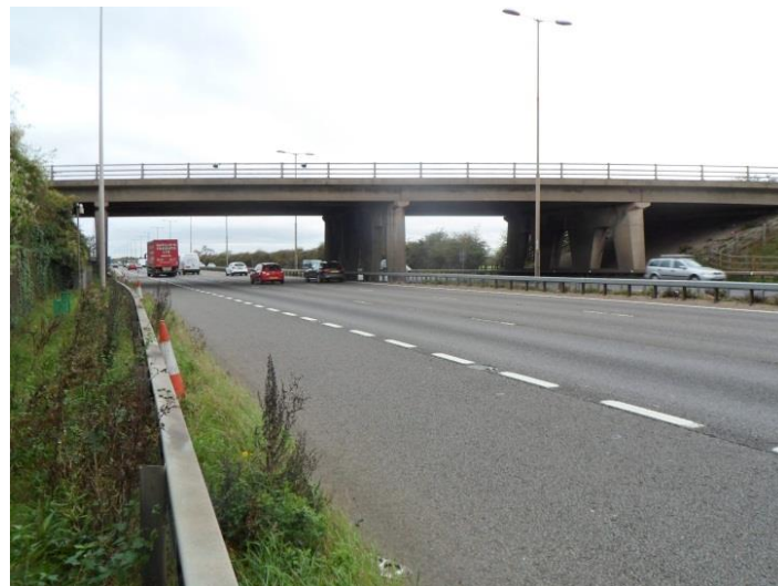
Figure 5 View of Existing Lake End Road bridge
