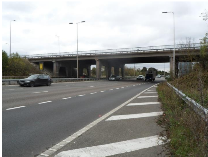
Figure 28 View of the existing Huntercombe Spur bridge
